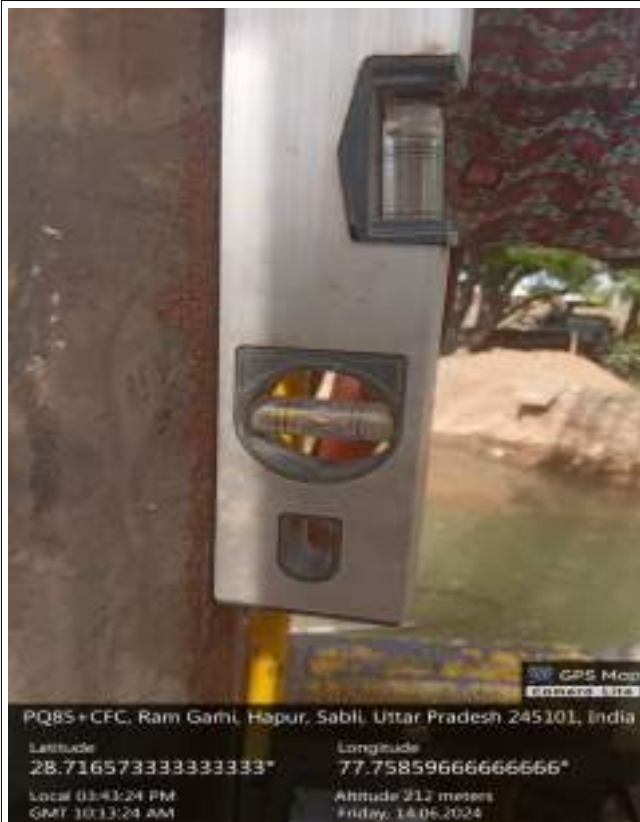
Fig 5: Level of lowering Pipe.
