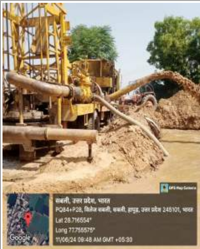
Fig. 03 – Drilling of Bore well.
