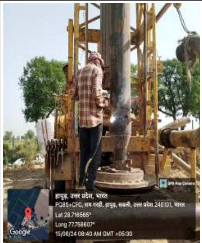
Fig 4: Welding of Lowering Pipe.
