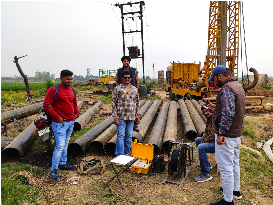
Photo of the Site at the time of Logging
