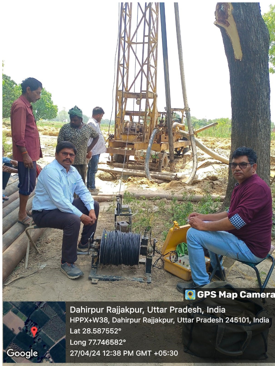
Photo of the Site at the time of Logging
