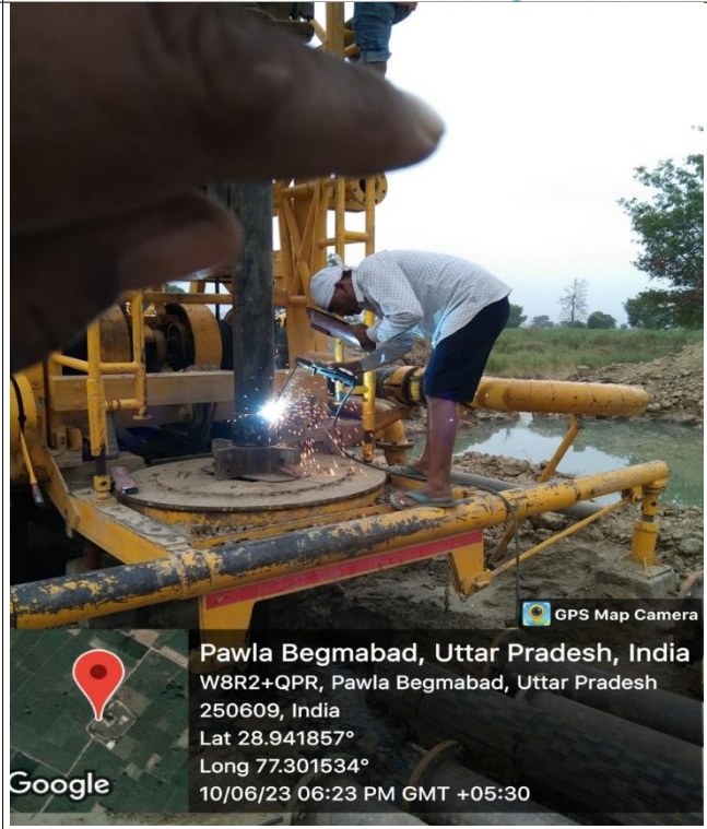
Fig 5 Lowering in progress.
